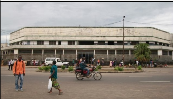
Original view of Pax Polyclinic in Kananga, as seen from the front.
