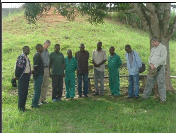
The hydro team prays in February, as they start the last day's work to see if two years of work on generator #2 will turn on and function!
